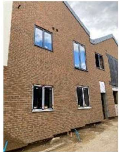
1200 x 1155 Tracker Panels for 65mm brick Slips 3mm Deep with 10mm Mortar Joints
